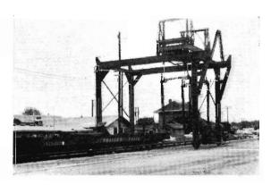
Straddle type crane used for loading semi-trailer container units and containers.
