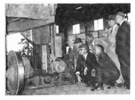
Watching the bogies of a wagon being exchanged at Dynon.
