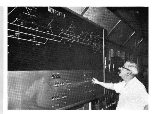
REMOTE CONTROL: Signalman P. McMahon makes a road on the new panel installed in Newport A signal box. On October 22, the single line between Altona Junction and Altona became automatically signalled, with the signals at Altona Junction controlled from Newport A Box.
