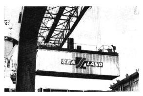
35-ft. Sea Land Containers being loaded onto ship at Elizabeth, New Jersey. Note special frame that is attached to top of container for lifting.
