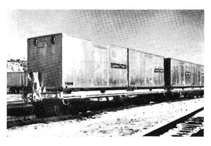
20-ft. container for Canadian National Railways. Note side doors: when the containers are left on the wagon to form a conventional box wagon, access is by way of these doors. However, they are too small for most fork-lift trucks, and, because they weaken the side of the container are not favoured by most operators in U.S.A.
