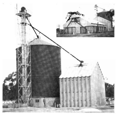
Wheat is received at the steel elevator (left), and passes to the Behlen shed used as an annex bin. Inset shows the oats storage bin adjacent to wheat storages.
