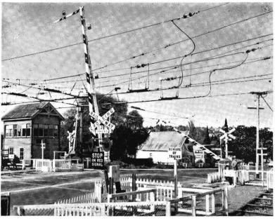
These barriers at Riversdale Road have arm tips that turn down to clear the tramway wires. There are four 27-ft. long arms—two on each side of the road. The installation of these barriers allowed the road to be widened from 29 ft. to 45 ft. They are controlled by the signalman at the crossing.
